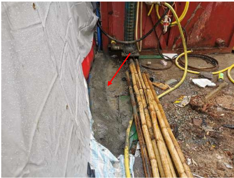
Figure A2 Rectification by Contractor- Small concrete bunds provided along the site boundary in Zone D3
