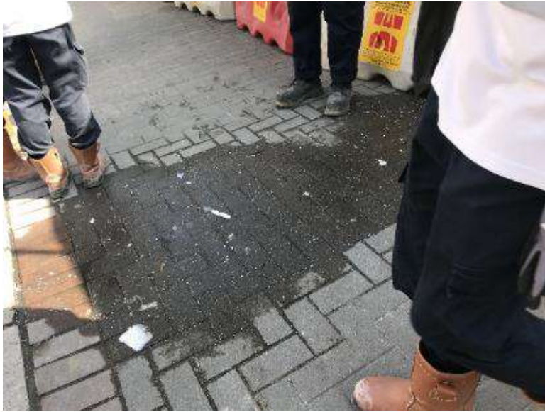
Figure A1 Observation on 4 February 2021 in Zone D3- Site runoff from flowing out of the site boundary in Zone D3
